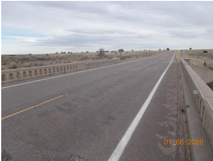
View of bridge M-21-B looking northeast.
